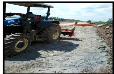
Mixing with in-situ soil
