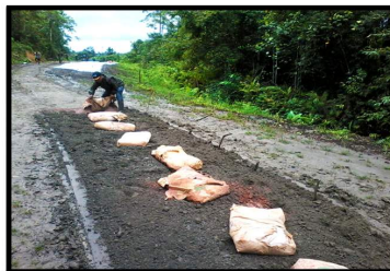
Spreading of TF - 40 kg bag
