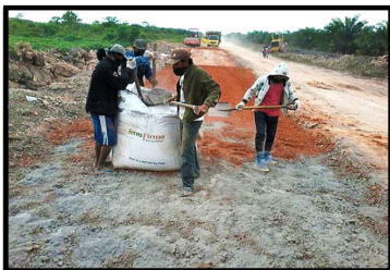
Spreading of TF - 1 jumbo bag
